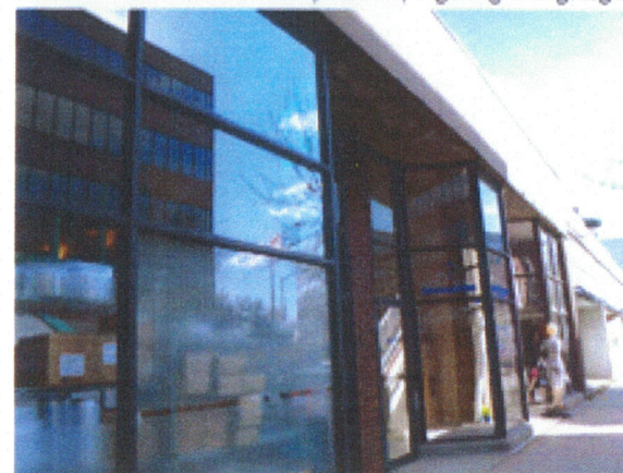
Sidewalk Storefront Soffit and Fascia
