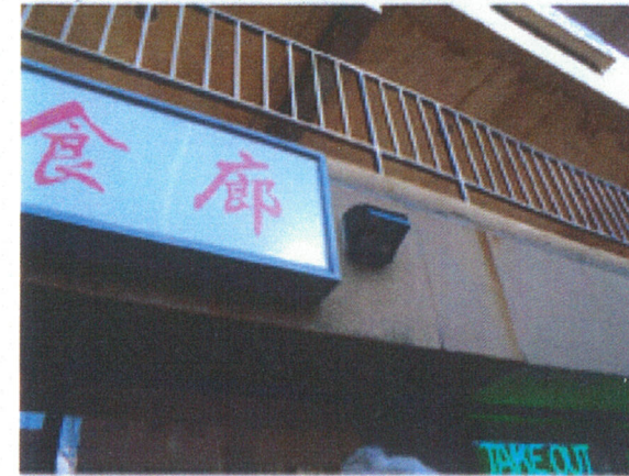
Lower Level Terrace Soffit, Fascia, Lighting & Signage
