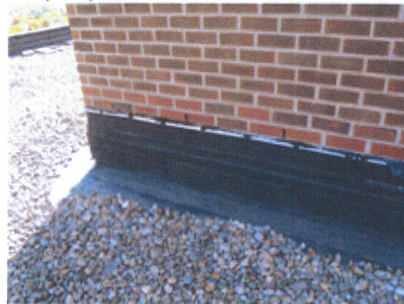
Counterflashing at Masonry and Roof
