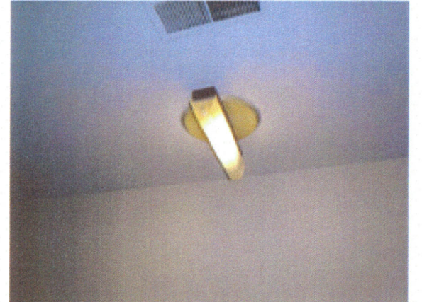
Hallway Ceiling with HVAC Register and Light
