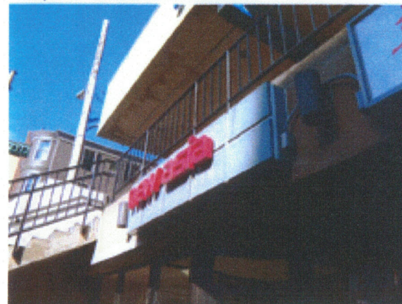
Fascia, Lighting and Signage at Stair
