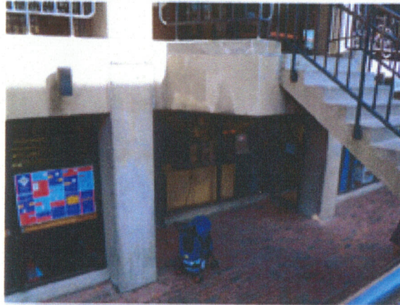
Lower Level Terrace at Stair
