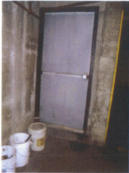
Garage Exit Door to Street
