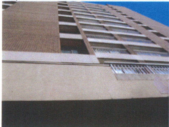
Tower Masonry Cladding, Fascias and Rails
