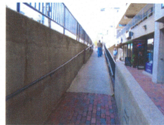
Ramp from Sidewalk to Lower Terrace
