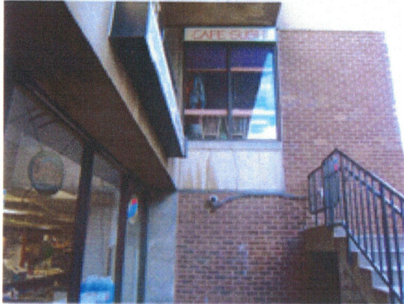
Storefront Masonry Cladding, Soffits and Fascias
