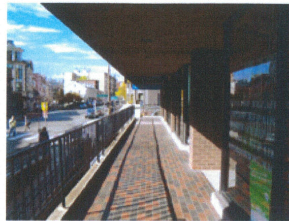
Entry Level Terrace Looking Northwest
