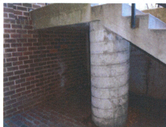
Step Support at Terrace Southeast End
