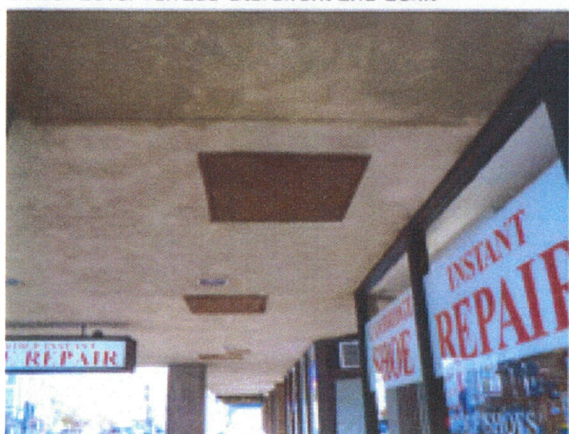
Upper Level Soffit and Signage Detail
