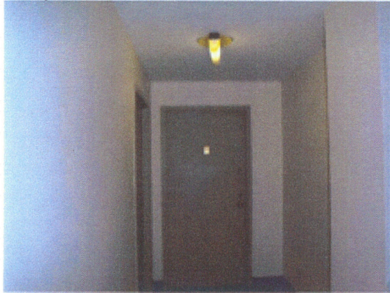
Typical Hallway Doors
