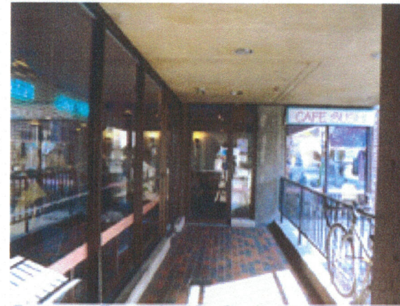
Entry Level Terrace Looking Southeast
