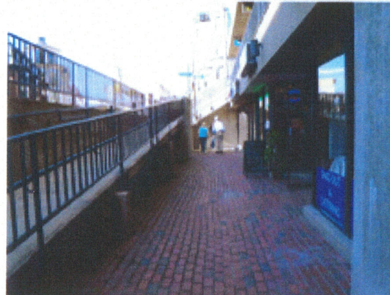
Lower Level Terrace at Ramp Looking Northwest
