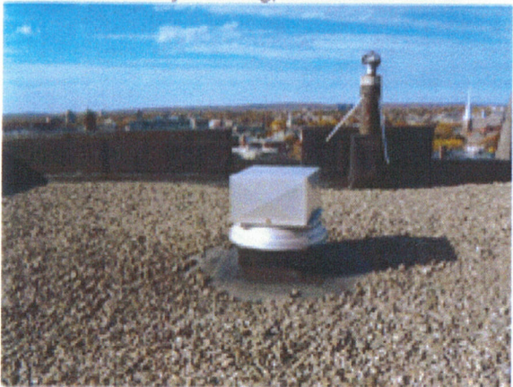
Rooftop Equipment, Ballast, & Parapet Flashing
