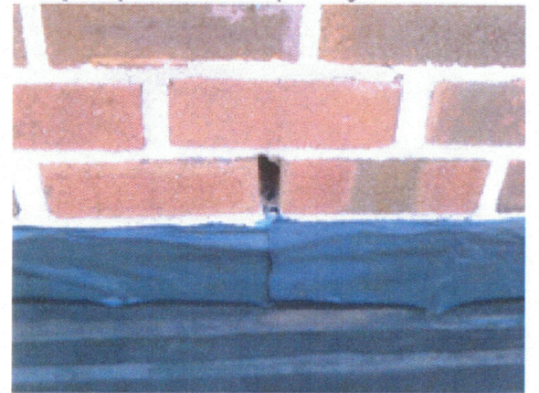
Masonry Weep Detail at Counterflashing
